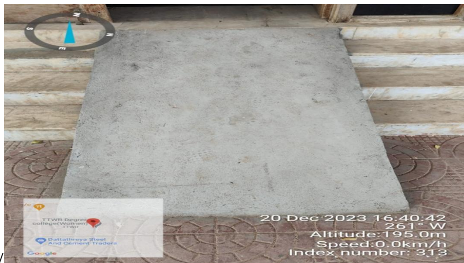
RAMP FOR DISABLED STUDENTS.
